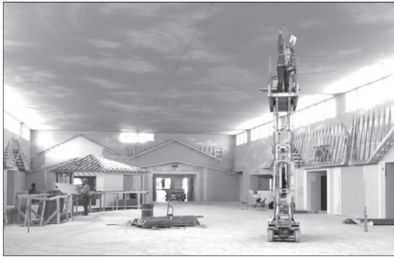
Using a lift, Lili Payne was able to reach a ceiling to paint a bird at the Thief River Care Center. By hand and, in some instances, with the help of machines, Payne created four murals and 123 window inserts for the new building. (Submitted)
